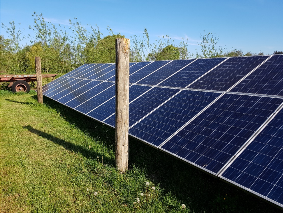
Figure 12: Pole placement for each PV-string
