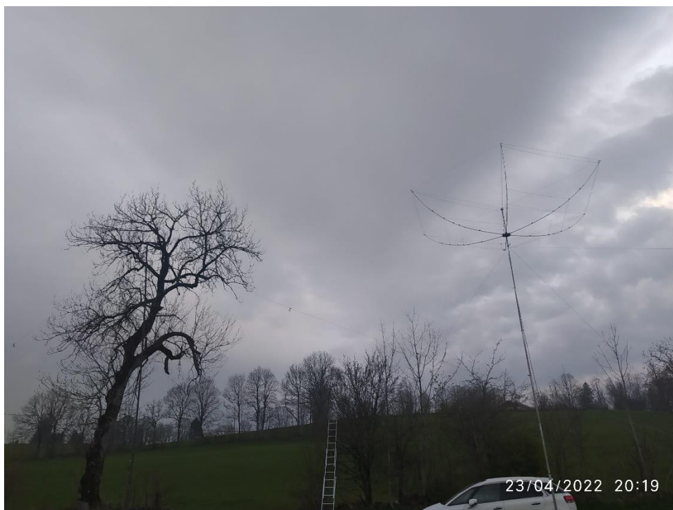
Inband antenna close up
