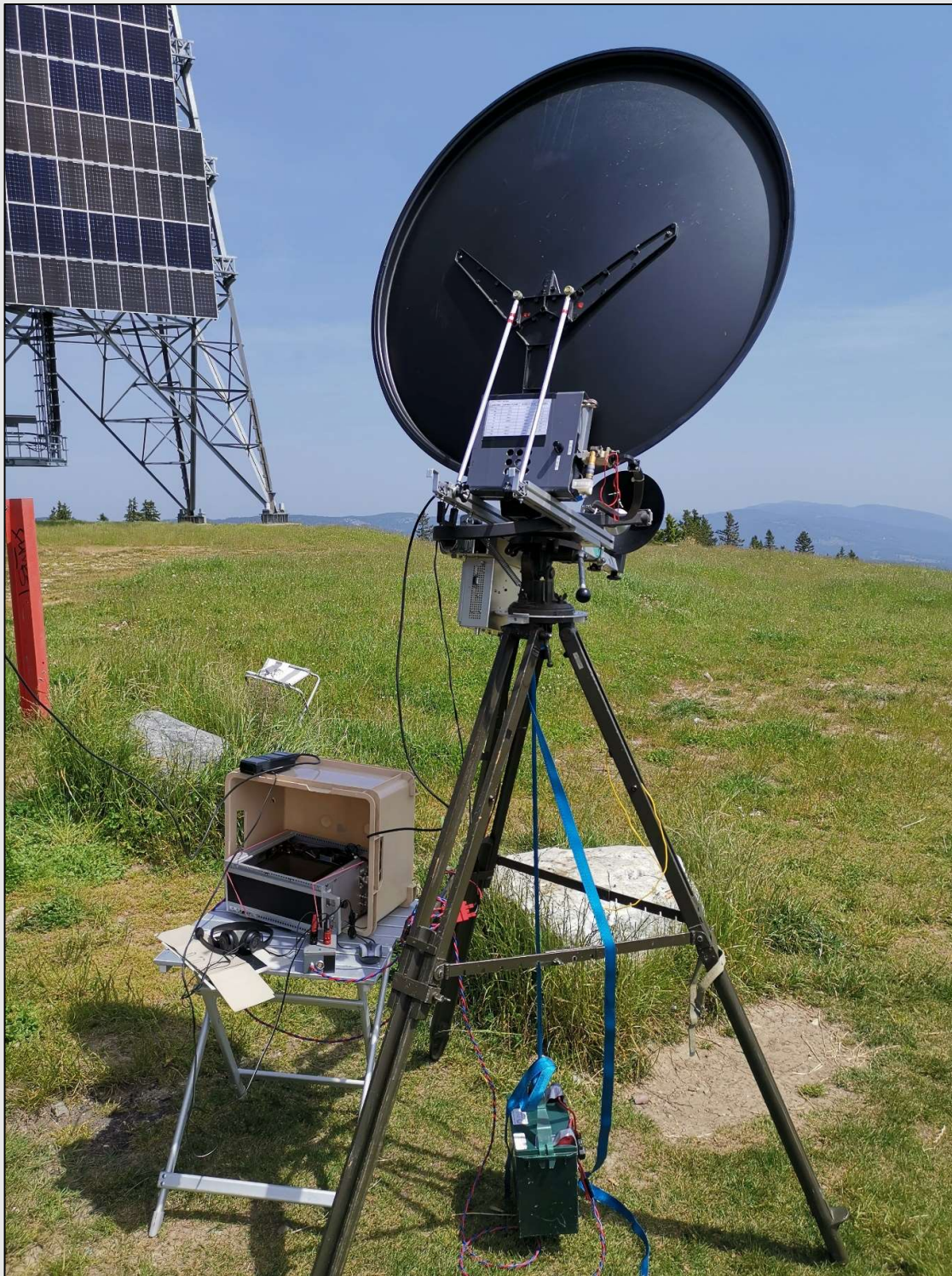
Station HB9DUG/p – QTH La Barillette (VD)
